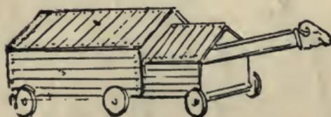
5. Battering ram with protecting cover, on wheels, called a "tortoise," from M. Rodios' work.
