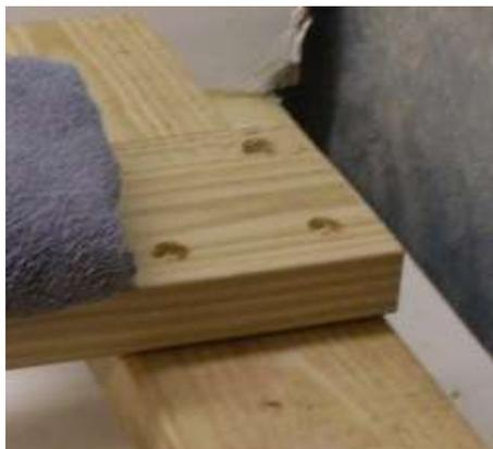
Counterbore the back holes on the top board and on the bottom side of the bottom board. This way the bolts will sit inside the wood and not stick out. Insert the 1/4 inch by 3 inch bolts through each hole and put a washer both top and bottom. No washers go between the boards. Screw these down tight and use a lock washer against the nut, and apply loctite if you have some.
